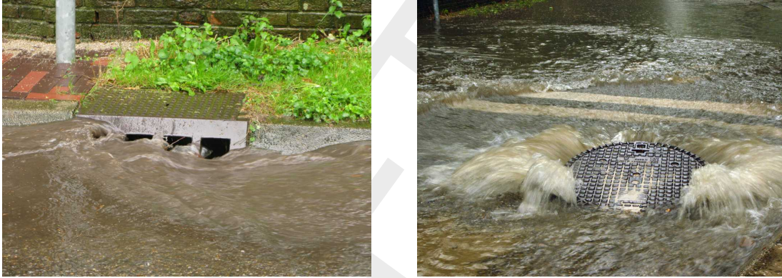
Figure 8.35: Examples uses for 1D2D vertically stacked connections. Left: street inlet. Right: manhole cover. (Source: GAW/Stichting RIONED)
